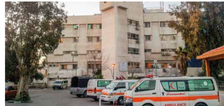
The exterior of Al-Shifa Hospital, the largest and busiest healthcare facility in Gaza
